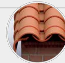
Edges clay accessories are installed so that they are always underneath the covers that form each side, and in the same direction as the pan curved roof tile.
