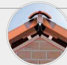
The Under ridge roll tape (mixed, aluminium or Roof ridge pvc vent brush) should be placed on the ridge batten and fixed with clips or nails. The rolls have adhesive strips of butyl to attach to the profile of the roof tiles and waterproof joints. Finally, the Ridges and End Caps clay accessory should be installed with screws/ nails and ridge clips.
