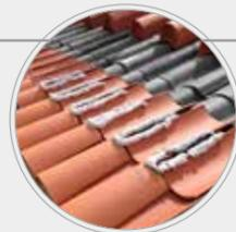
Structure with under-tile Corrugated bitumen sheet or Fiber cement sheets. Follow Guide for installation in force for these products.
